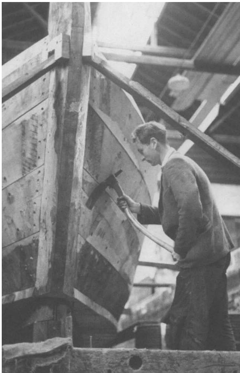
8. A boat builder using an adze to complete the shaping of a stem post.
